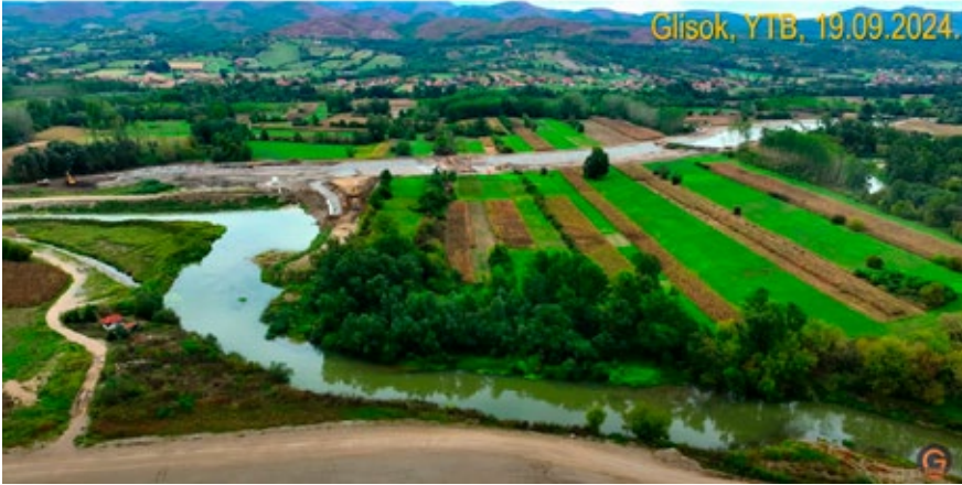
Construction works on meander cut-off on the Zapadna Morava River
